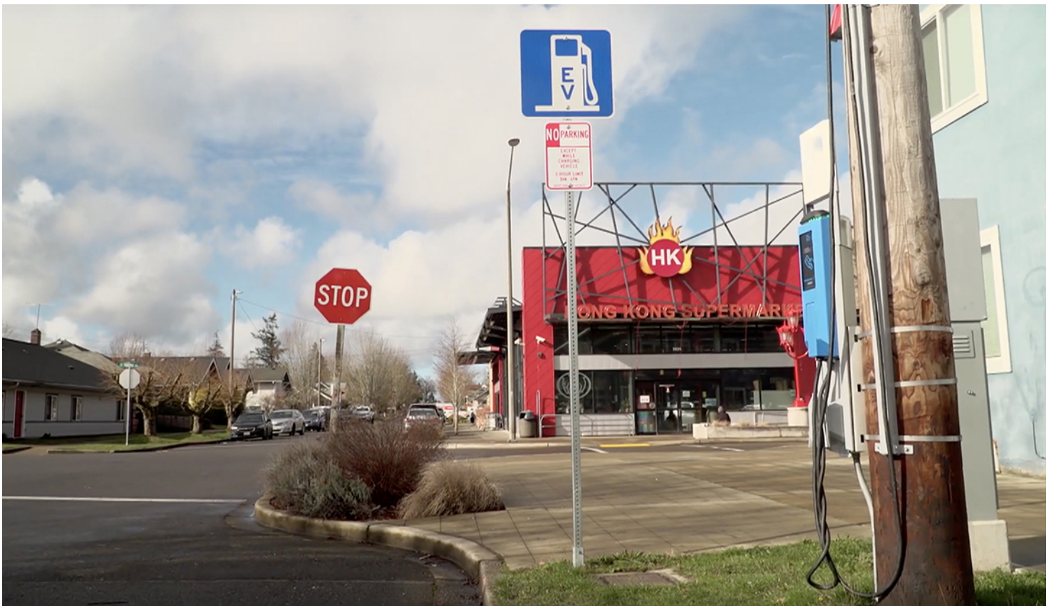
Tacoma, Washington's 15 neighborhood business districts each have received one new streetside charger, according to a City of Tacoma video . The chargers are affixed to energy-efficient LED streetlights, freeing up electricity to support the chargers with minimal upgrades. Photo courtesy of City of Tacoma.
