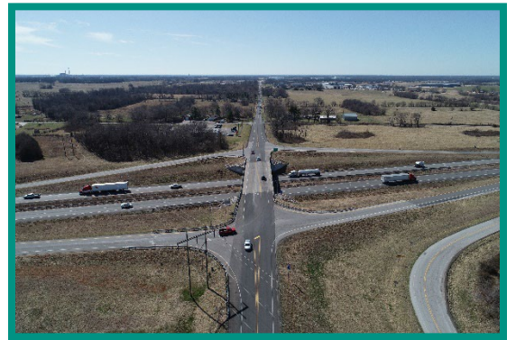
Figure 3 Hwy MM Bridge over MO
