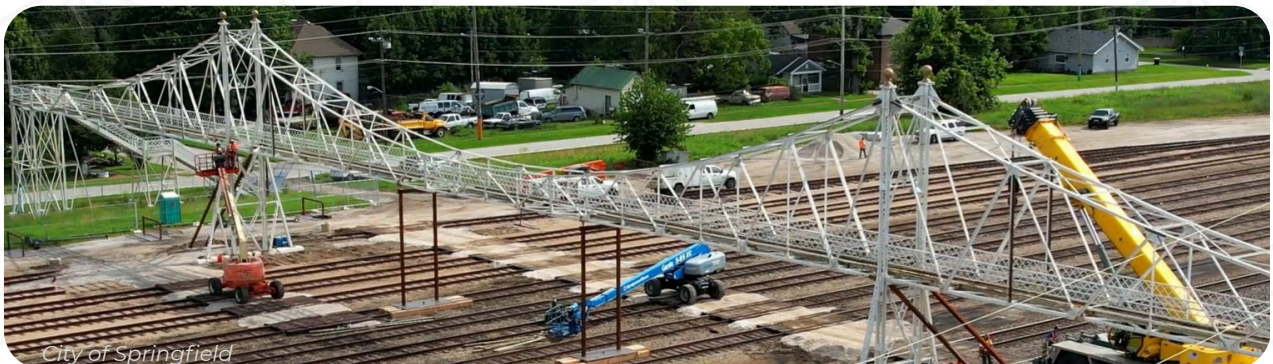
Jefferson Avenue Footbridge Disassembly
