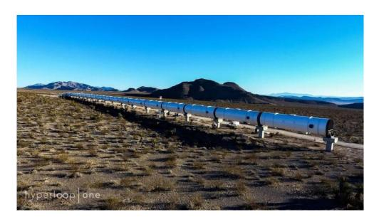
Hyperloop uses electric propulsion to thrust pods through a tubular track at high speeds. The pods could have screens with augmented-reality capabilities. HYPERLOOP ONE
