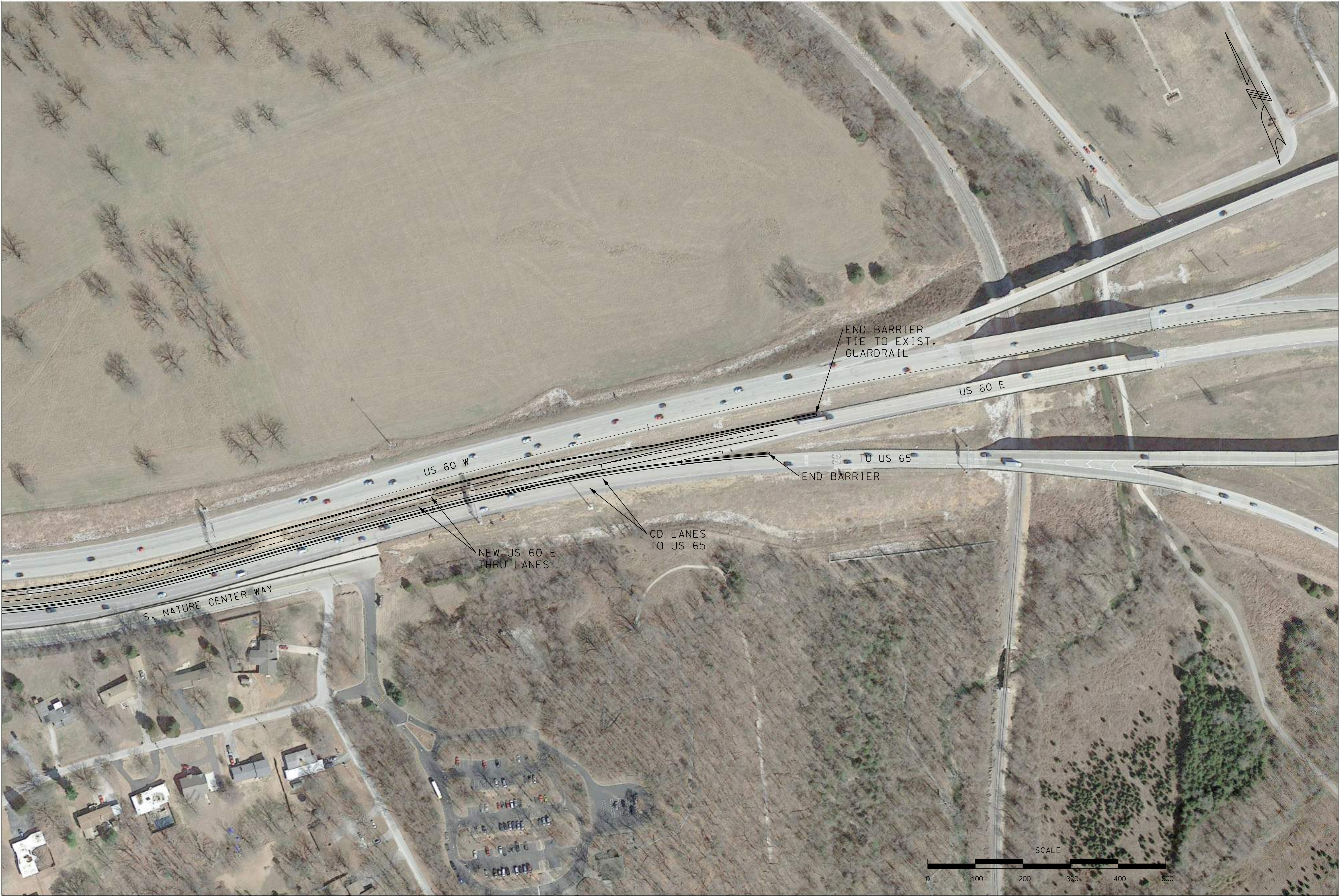
J8P3032 / US-60 - GLENSTONE INTERCHANGE
