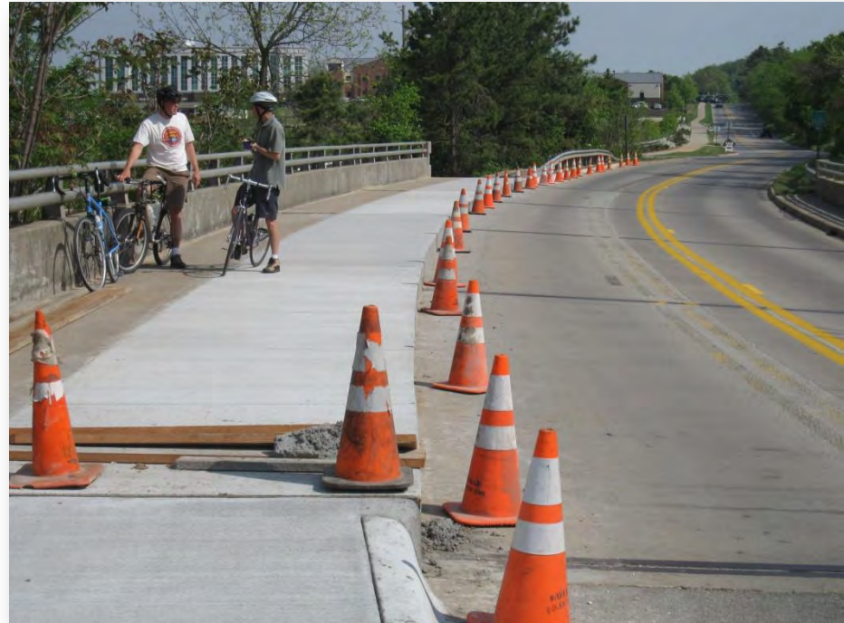
Figure 49 - Example of Narrowing Traffic Lanes to Provide Path on Bridge, Calm Traffic
