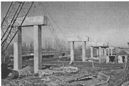
Setting the supports for the Miami Bridge.
