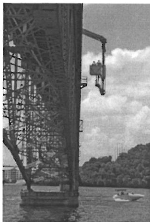
Inspectors examine the underside of the Hurricane Deck Bridge using a snoop truck.
